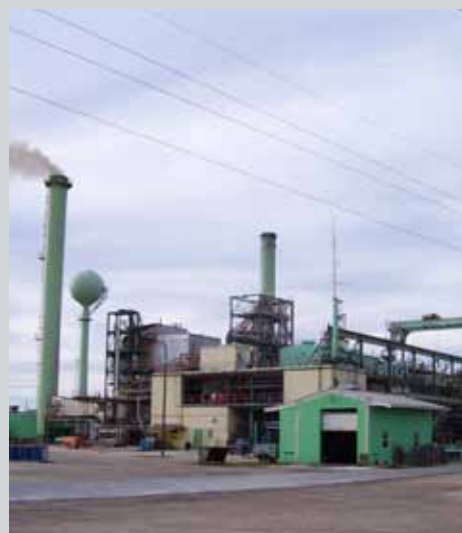
Grand Bahama Power Station
