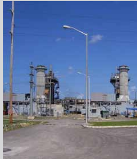
Bogue Power Station
